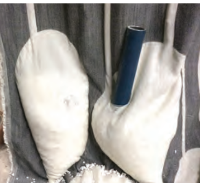
Figure 228: The process of filling the pockets with perlite using a tube.
